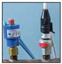
High-pressure safety high pressure transducer
